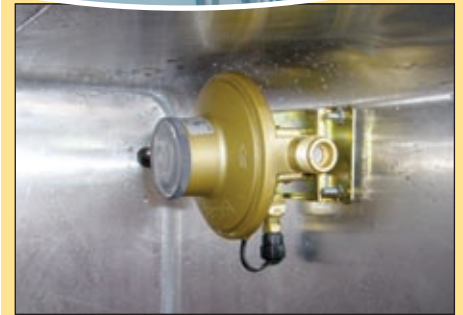
Typical Avondale configuration with Regulator in top right and inlet facing you.
