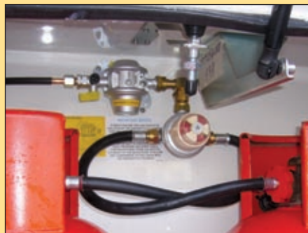
Option 2 Fit an 01-1755 automatic changeover head.
