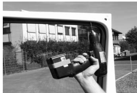
B25: Bore the holes which have been transferred into the door frame (Ø2.5 mm).
