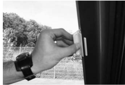
C2: To open: Loosen handle from rest position by tilting and pulling lightly. To close: Latch in handle by pressing onto cassette.
